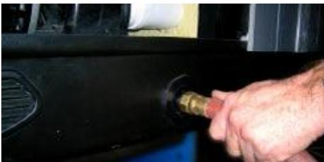
**Note:** The Spa will drain about 20 litres per minute. Ensure that the drainage is in an area safely away from window wells or basement entries.
